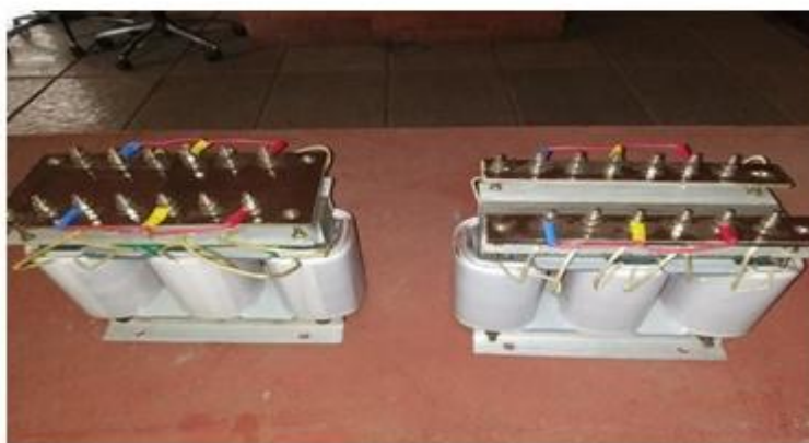
Fig.1 Healthy and deformed 3-Phase, 1KVA transformers
